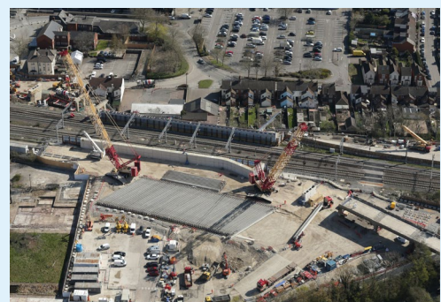
Over 100 beams wait to be installed on Bletchley Flyover
