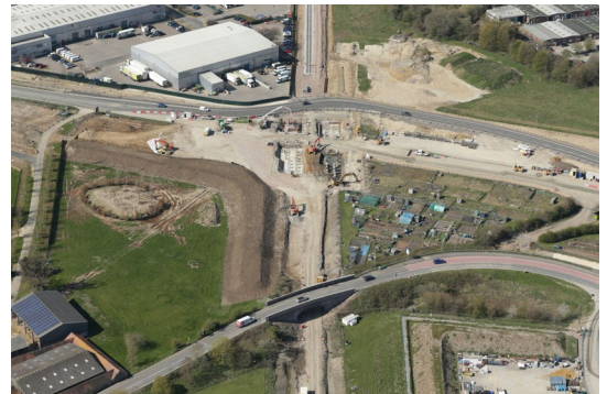
Charbridge Lane overbridge, April 2021
